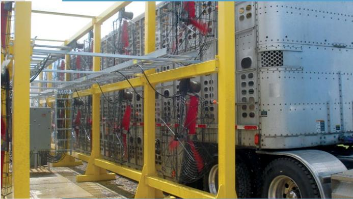
Combined water sprinkling and ventilation system.
