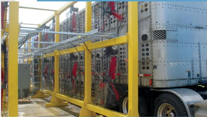
Combined water sprinkling and ventilation system.
